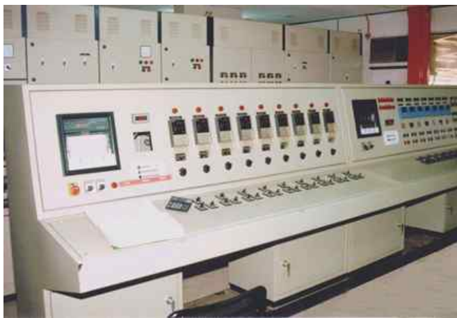
Central Control Panel
